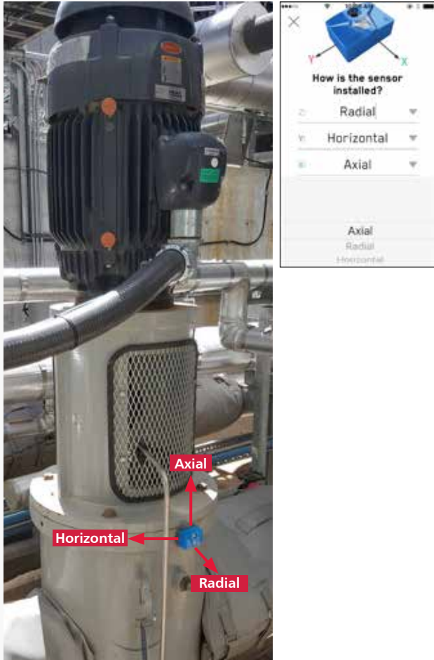
Figure 34: Standard orientation on a vertical pump
